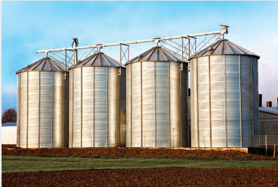
Fig. 22-28: The gas formed during fermentation of crops stored in a silo can kill within minutes when inhaled. Photo: © Shutterstock.com/Jorg Hackemann.
